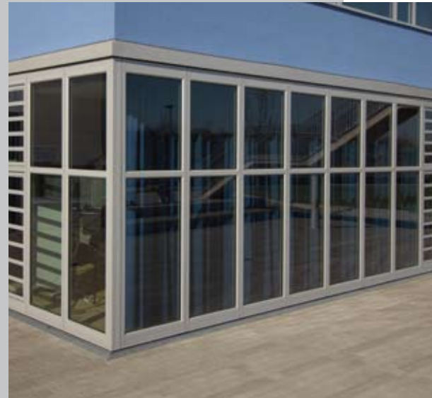
The façade of a music room closed with Thermoflex. Lamellar windows are integrated for ventilation.
