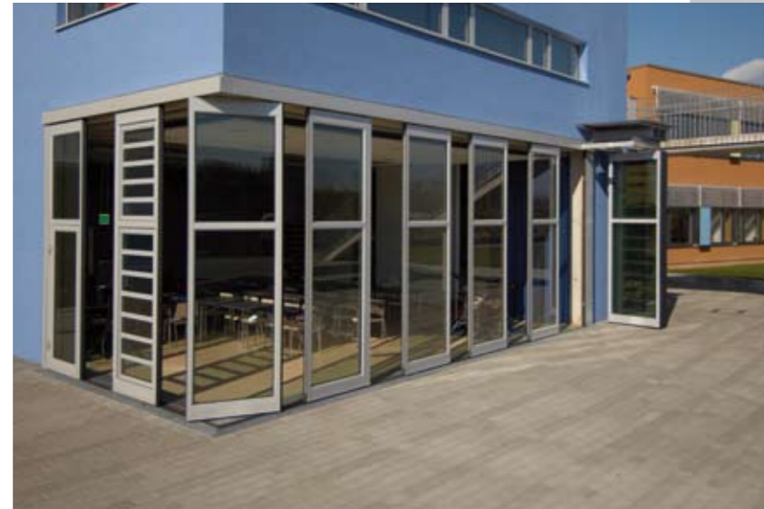
The mobile Thermoflex elements are detached, manoeuvred over the 90° corner and positioned outside of the wall pivot.
